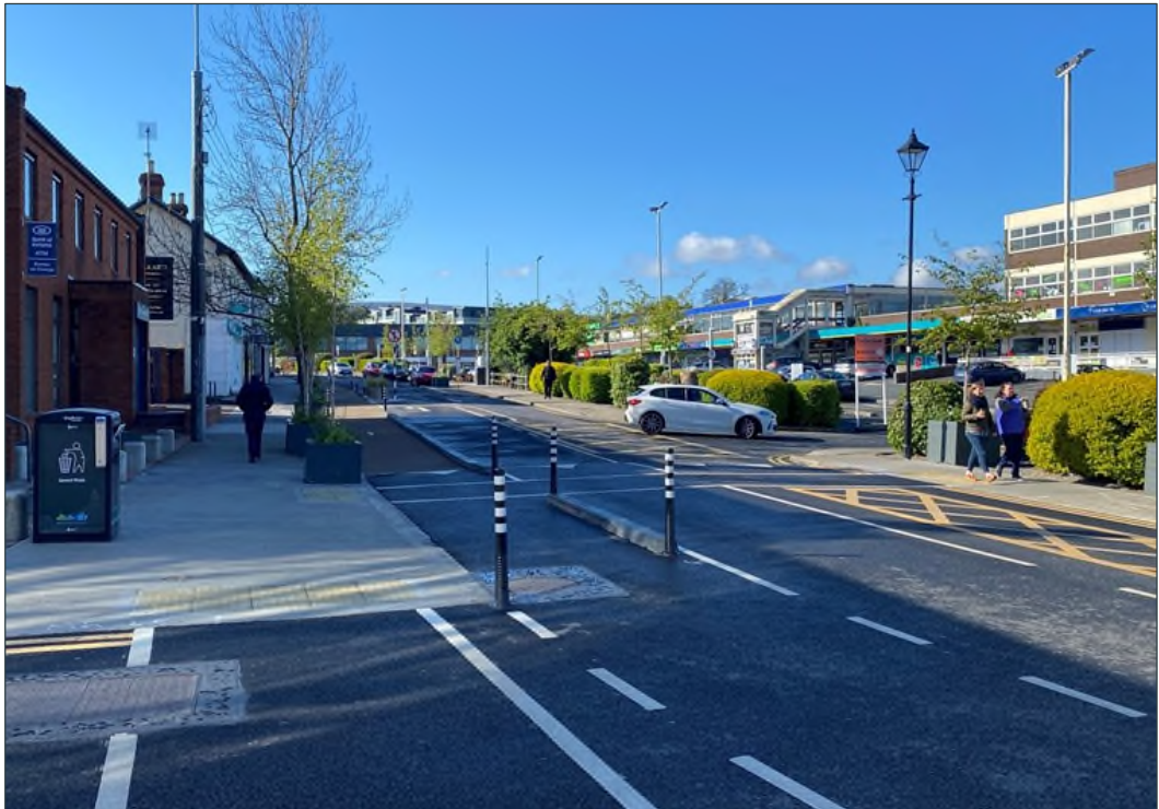
Figure 3.3: Existing Pedestrian Crossing at Main Street
