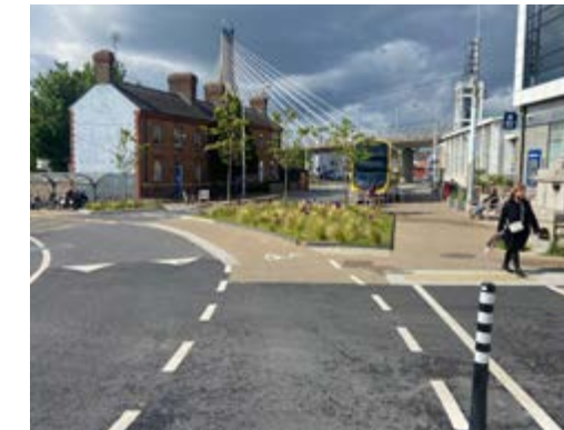
View from Main St. towards Luas bridge
