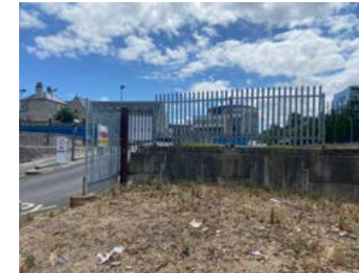
Retaining wall with railings on top
