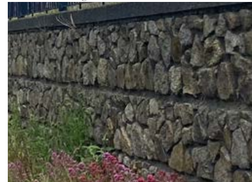
Existing Rubble Wall
