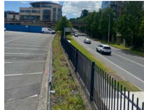
Retaining wall with railings on top
